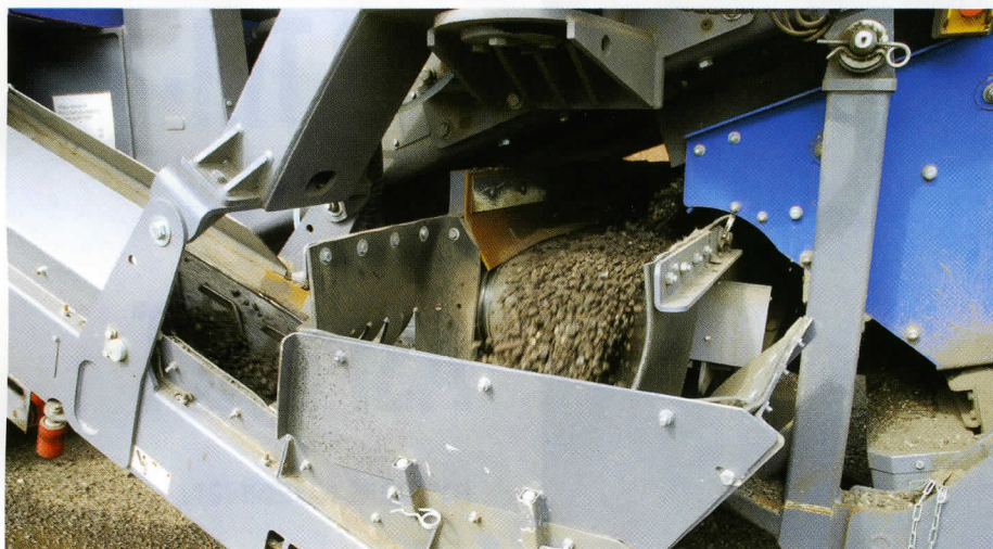
TOP: The final product out of the crusher is a minus 9/16-inch top size. Oversize material is initially returned for crushing. BOTTOM: The asphalt plant is located in a relatively small urban footprint adjacent to an interstate highway interchange, immediately southeast of downtown Youngstown, Ohio. The mobile crusher had to fit into the tight space.
