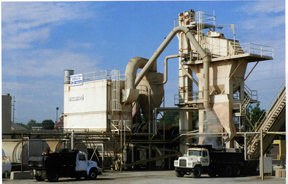
ABOVE: Tri-County Asphalt’s Stansteel batch plant produces about 160,000 tons per year. The company serves predominantly commercial customers with a variety of mixes; about 80 percent of production is destined for private sector use. LEFT: Much of the recycle coming to the Tri-County Asphalt Materials site is in the form of millings, but the material comes from many sources. As this raw RAP stockpile shows, proper screening and crushing is necessary to achieve consistent RAP feed for mix production. Plant Manager Chuck Royer said that’s especially true with state work.
